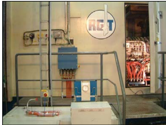
LM2500 Gas Turbine
